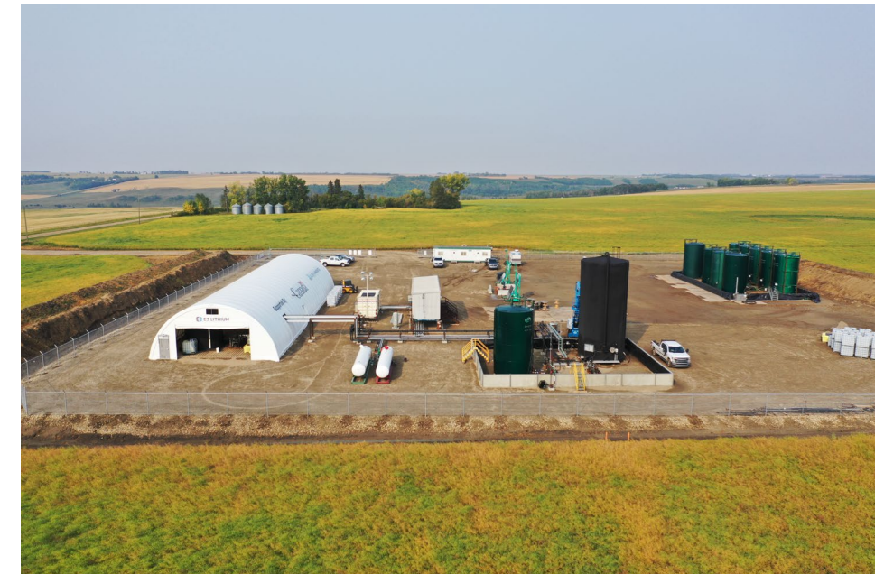
E3 Lithium’s field pilot plant in central Alberta was constructed and operated in 2023.
